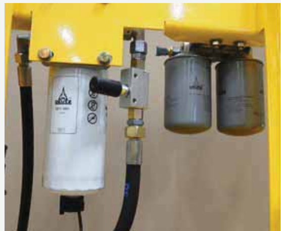
Multi-stage fuel filtering.
